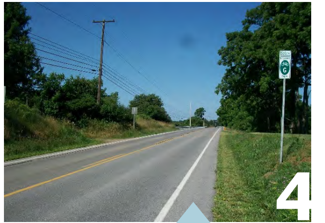
Least preferred are state or locally designated bicycle or pedestrian facilities on roads with narrow shoulders.
